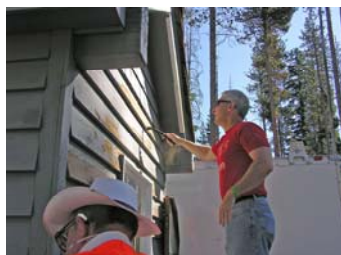
Craig Ackerman, Park Sup't, scraping old paint off.
