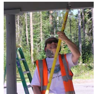
Judy Buckingham painting underside of entrance station overhang.
